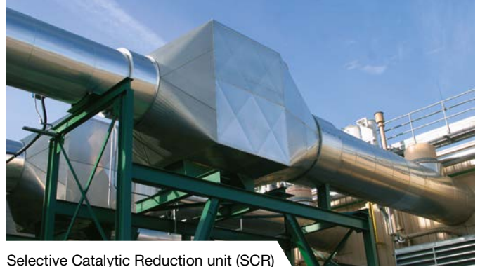
Selective Catalytic Reduction unit (SCR)
