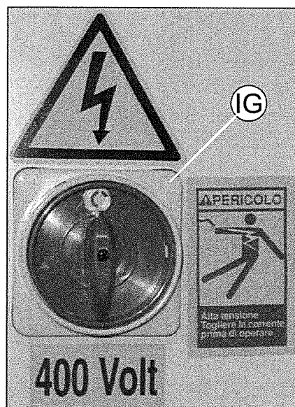
Fig. 4.3 Cut-out switch
